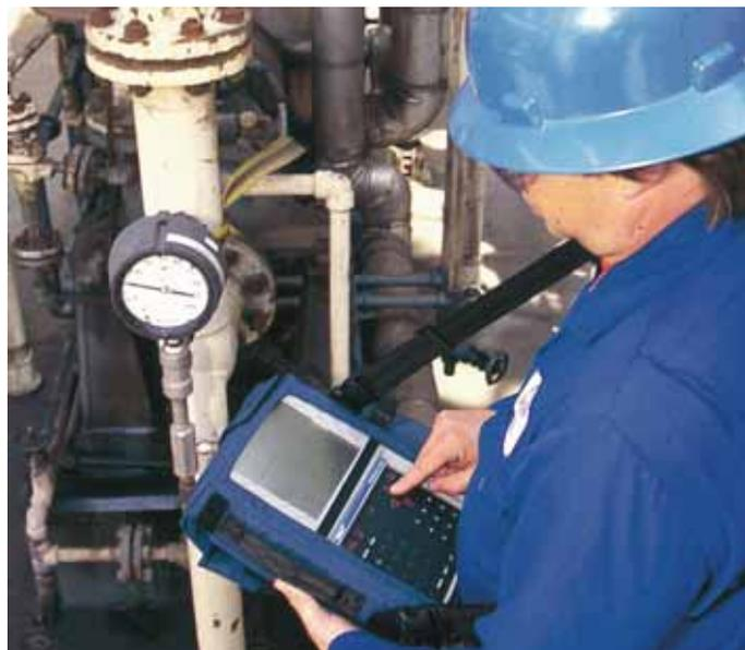
*Microlog® – portable data collector and analyser*
